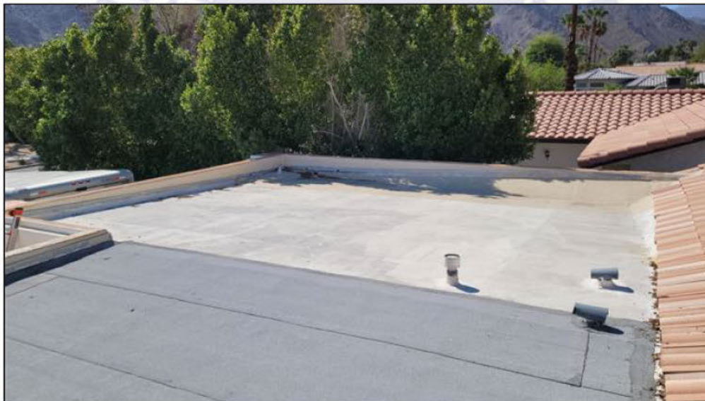
Low slope roof view
