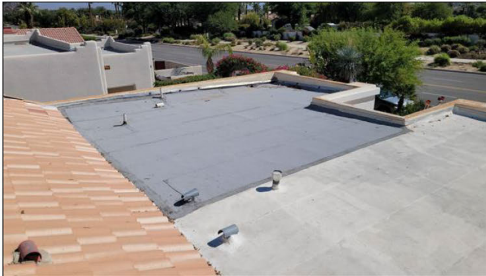
Low slope roof view
